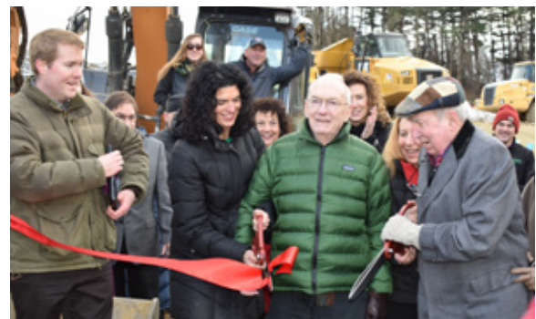
Brothers Dan and Leo O'Brien cut the ribbon celebrating the project commencement.
